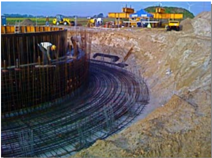
Excavated raft foundation of wind turbine
